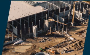
New Build & Plant Relocation
