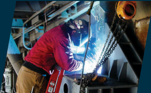
Emergency Repair & Maintenance
