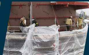
Alternate Access & Scaffolding Solutions
