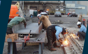
Onsite Machining & Fabrication
