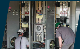
Electrical/Controls Design & Installation
