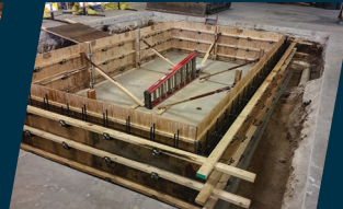
Foundations & Civil Construction
