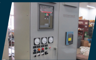
Retrofit, Upgrade, & Troubleshooting
