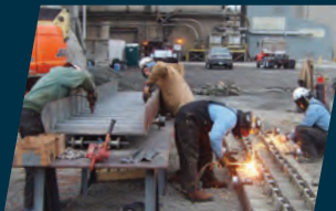
Onsite Machining & Fabrication
