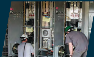
Electrical/Controls Design & Installation
