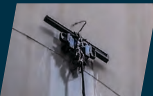
Onsite NDT Testing & Inspection
