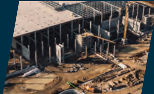
New Build & Plant Relocation
