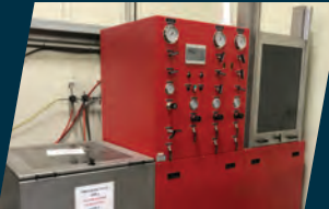
Hydraulic & Gaseous Pressure Testing
