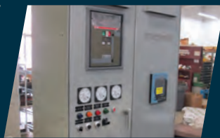
Retrofit, Upgrade, & Troubleshooting
