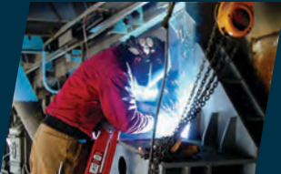
Emergency Repair & Maintenance
