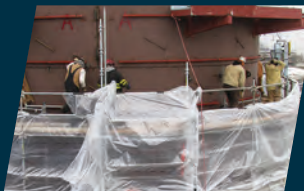
Alternate Access & Scaffolding Solutions
