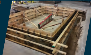
Foundations & Civil Construction
